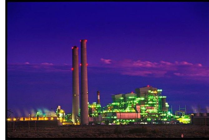
APS Cholla Power Plant,
