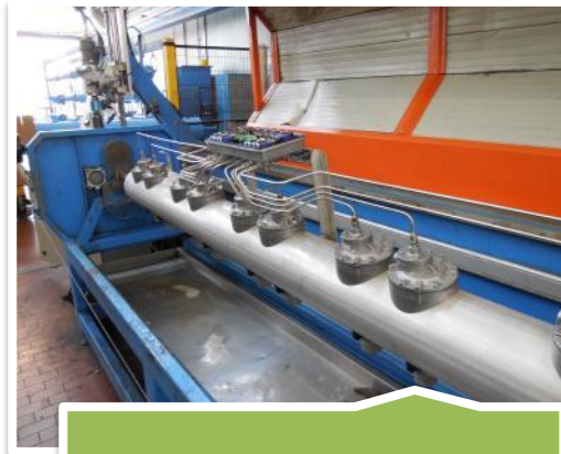
Pressure & leak testing
